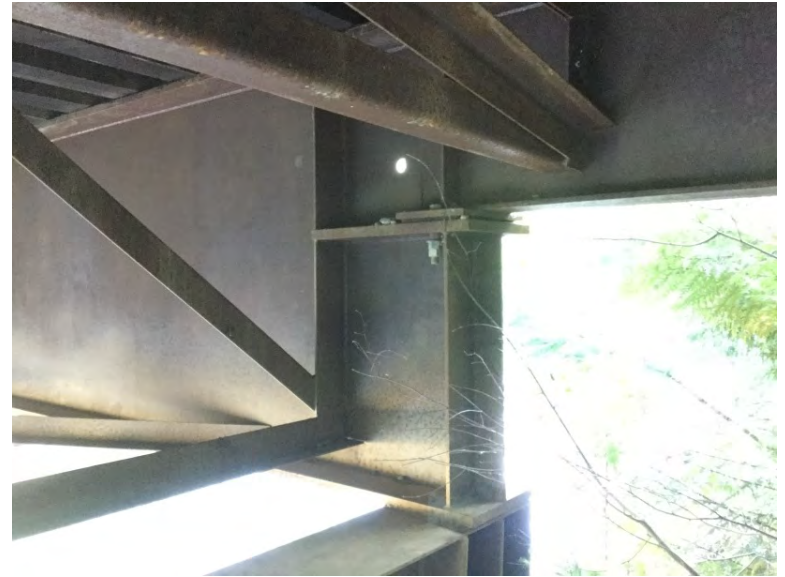
Main span to jump span connection
