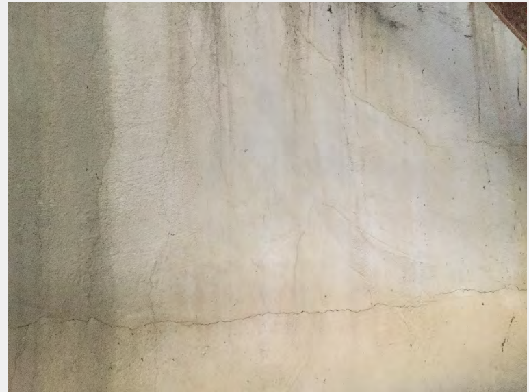
Left bank ballast Wall Condition
