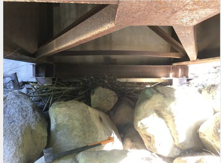
Left Bank Bearing
