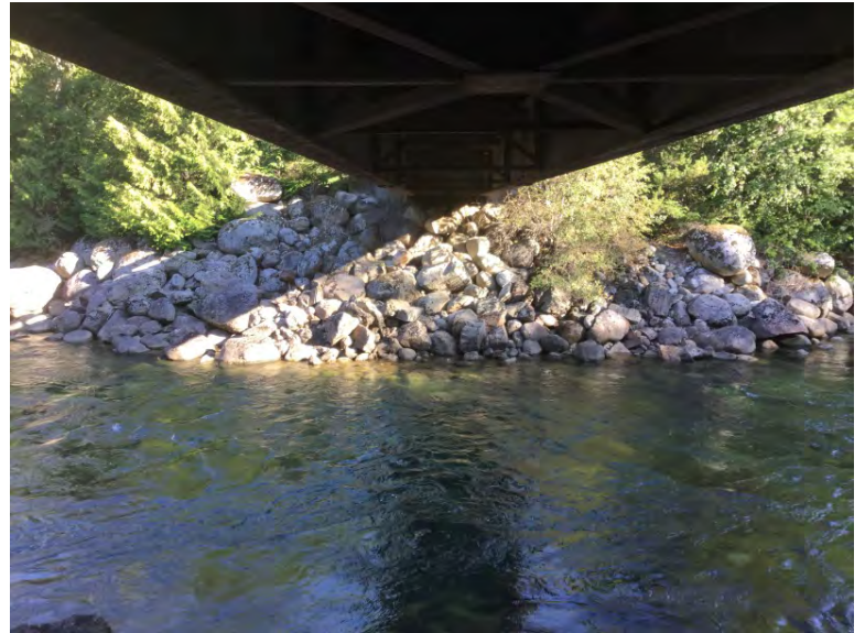
Left Bank Abutment when facing downstream
