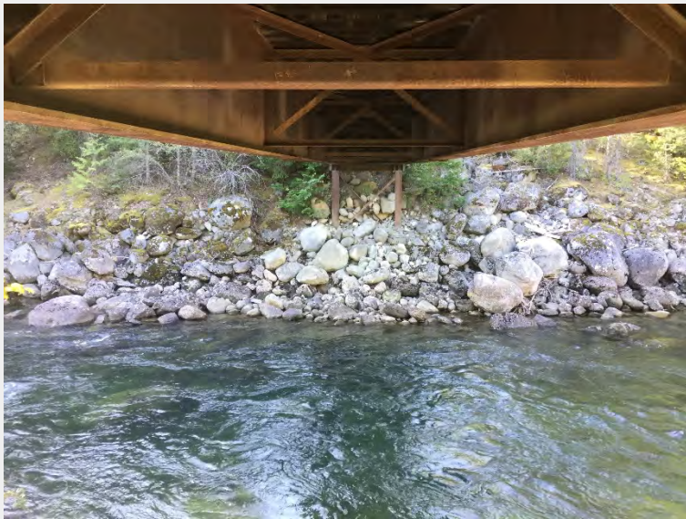
Pier and Right Bank Abutment
